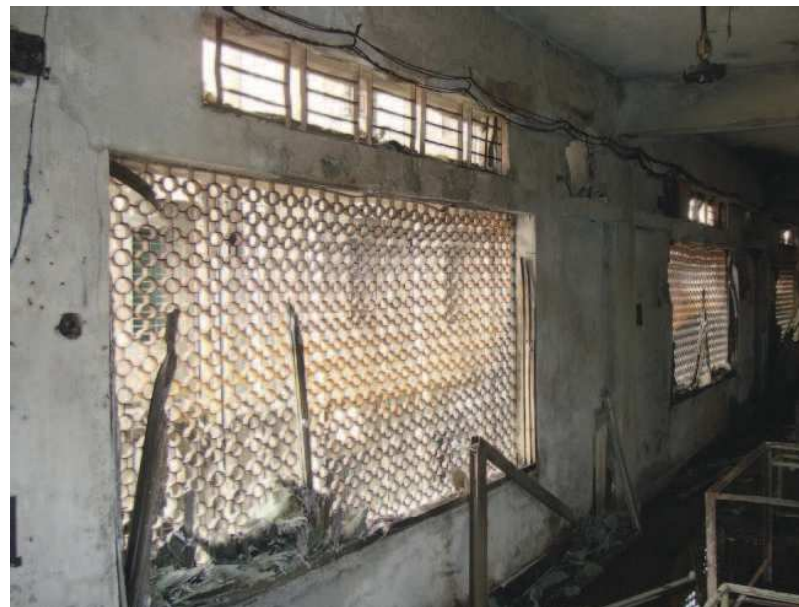
Broken glass in the Garib & Garib factory following the Feb. 25 fire.
