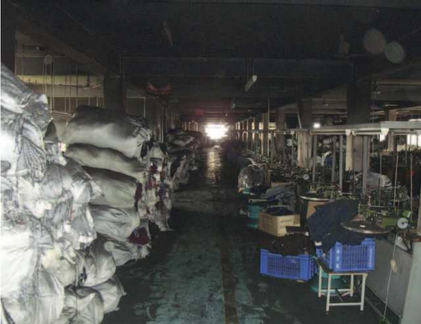
The fifth floor of the Garib & Garib Sweater Factory in Bangladesh is pictured above. A major fire in this factory on Feb. 25 killed 21 workers on the top floor.
