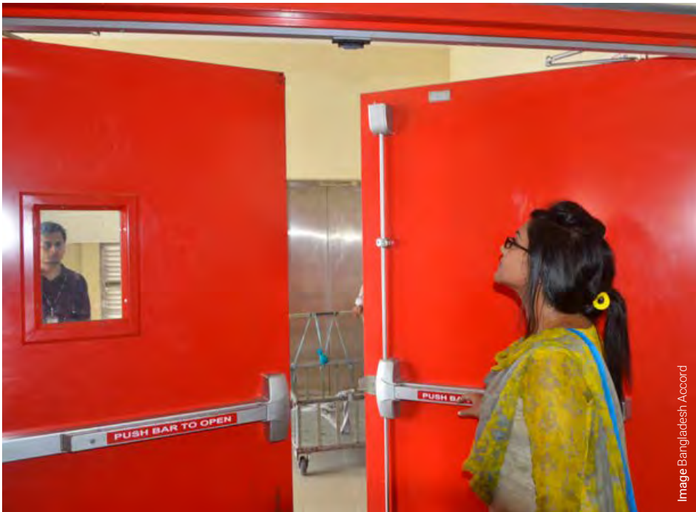
New fire-rated doors, installed in a factory covered by the Bangladesh Accord.
